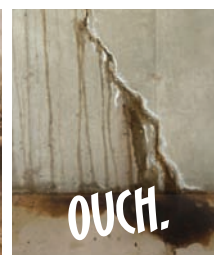
Wall Cracks
