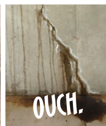
Wall Cracks
